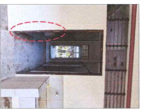
FRONT MALE CR DOOR JAMB NOTE: CHANGE TO CONCRETE DOOR JAMB AND CONSTRUCT NEW LINTEL BEAM
