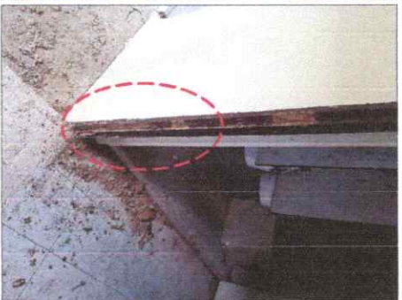
FRONT MALE CR DOOR JAMB NOTE: CHANGE TO CONCRETE DOOR JAMB AND CONSTRUCT NEW LINTEL BEAM
